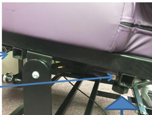
The arms are removable and / or adjustable for seat width. Each arm is supported on two square tubes which slide within two other square tubes. Each tube has a locking knob which should be tightened fully to secure the arm.
